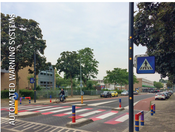
SMARTPOLE crossing installed including traffic lights, speaker and illuminated sign built into the column, designed to improve road safety for children near the local school.
