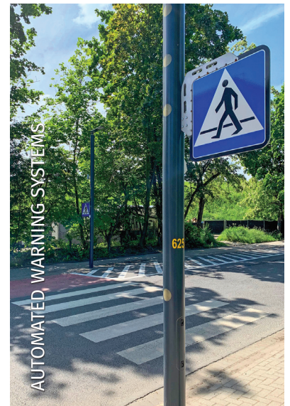
SMARTPOLE crossing installed to improve pedestrian safety. The column incorporates a warning signal, loudspeaker, illuminated sign and warning lights which activate when a pedestrian crosses the road.
