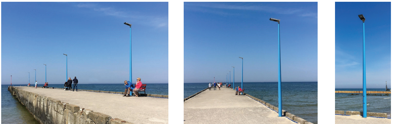
BASICPOLE installed in a coastal location. Finished in a sympathetic blue in order to blend into its surroundings.
